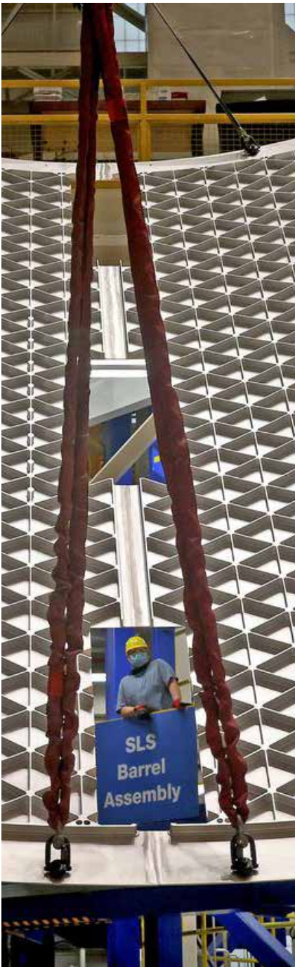
MAF_20210211_EUS_PanelLift01 (11 Feb. '21): Lift of three EUS test panels in VWC at Michoud Assembly Facility on Thursday, February 11, 2021. Technicians are manufacturing and testing the first in a series of initial weld confidence articles for the Exploration Upper Stage (EUS) for future flights of NASA's Space Launch System (SLS) rocket at the agency's Michoud Assembly Facility in New Orleans.
