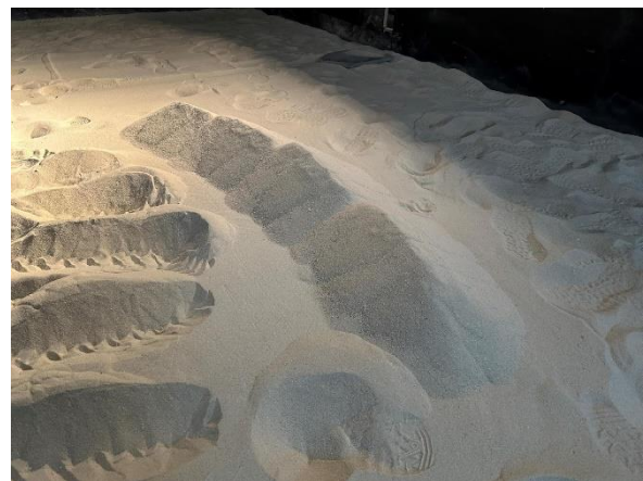
Figure 2. Fully constructed berm
