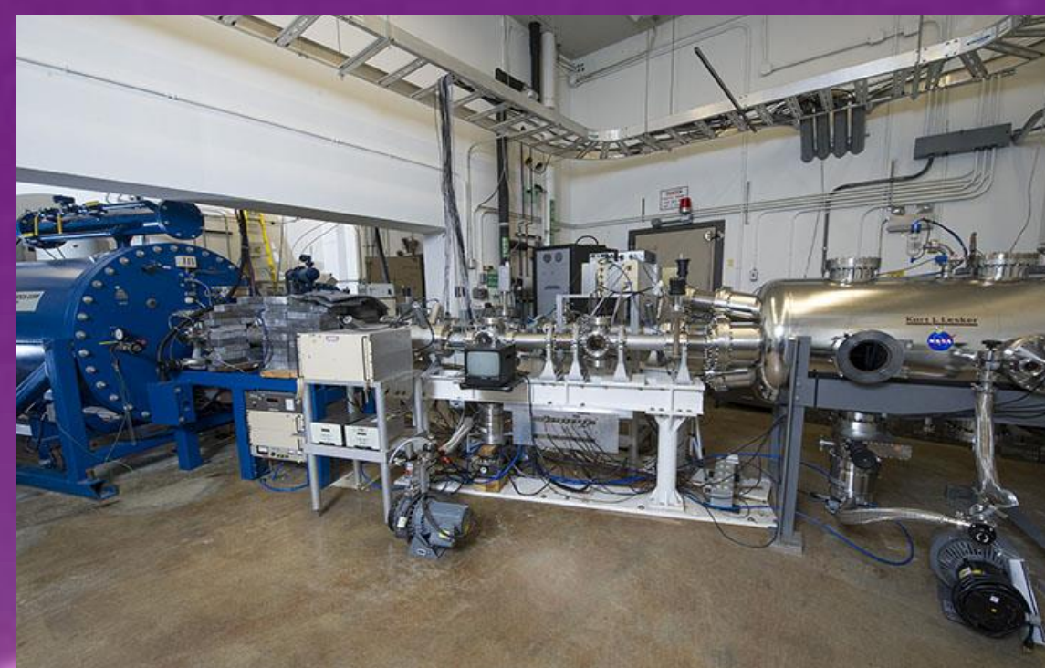
Side View of Pelletron beam line
